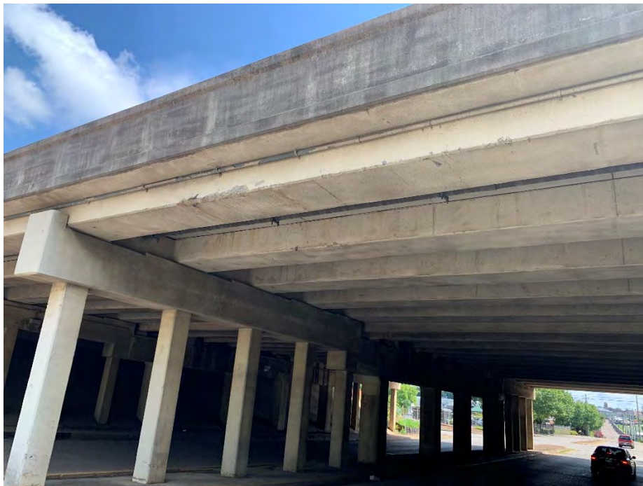
Damaged Beams Due to Impact Over Eastbound Lanes (Typical)
