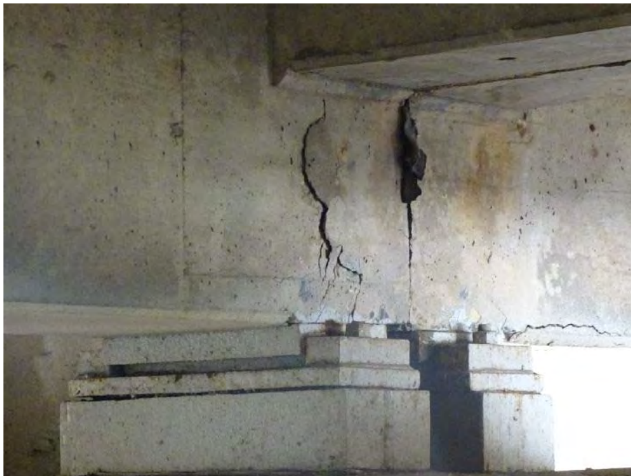
Spall on Beam Ends (Typical)
