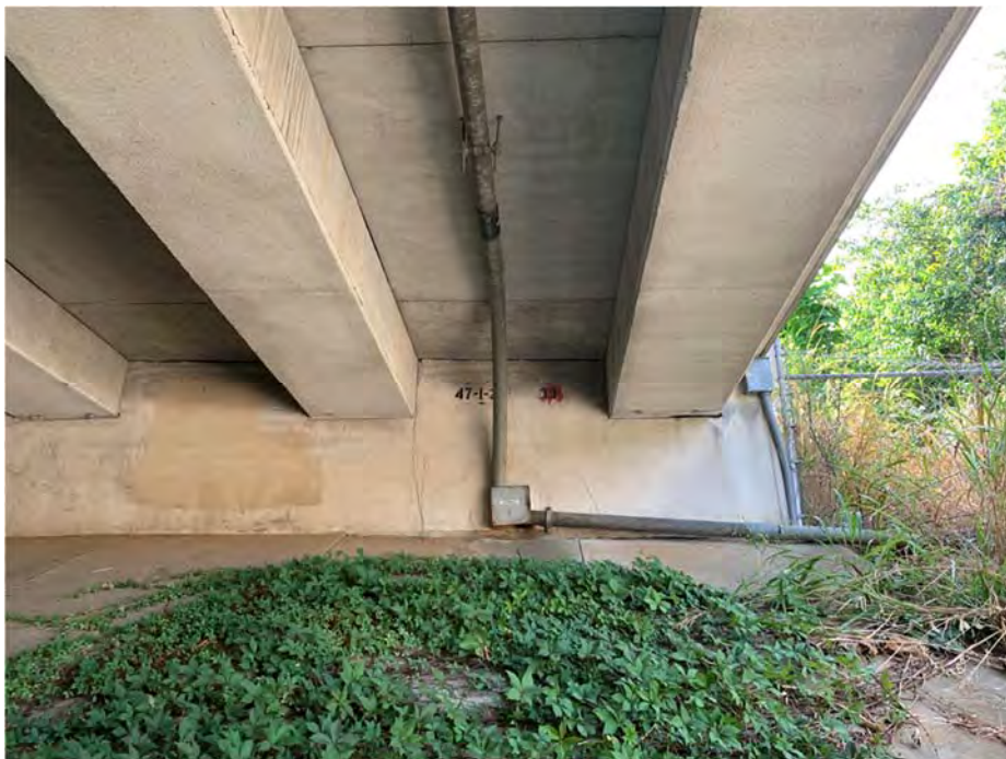
Mounted Conduit to Underside of Deck and Abutment No. 1 (Southwest Corner)
