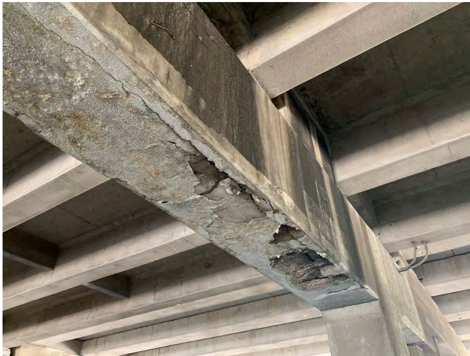
Spall on Bottom of Bent No. 2 (Typical)
