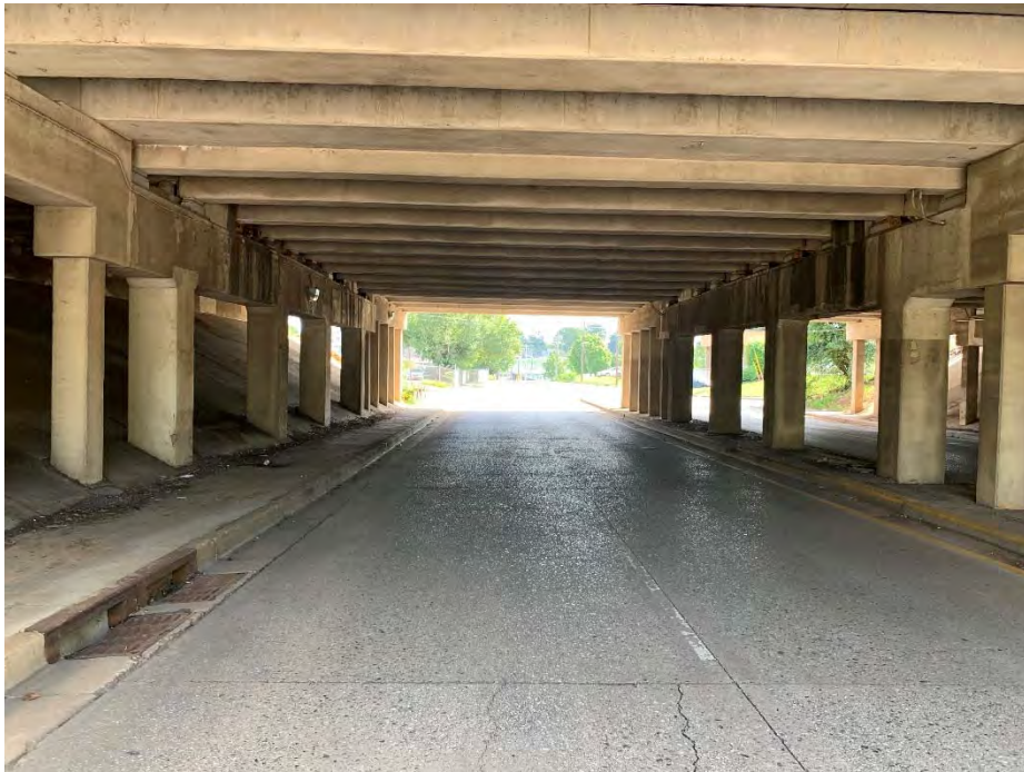
Span No. 3 Looking East Showing Conduit & Lighting Mounted to Bents (Typical)
