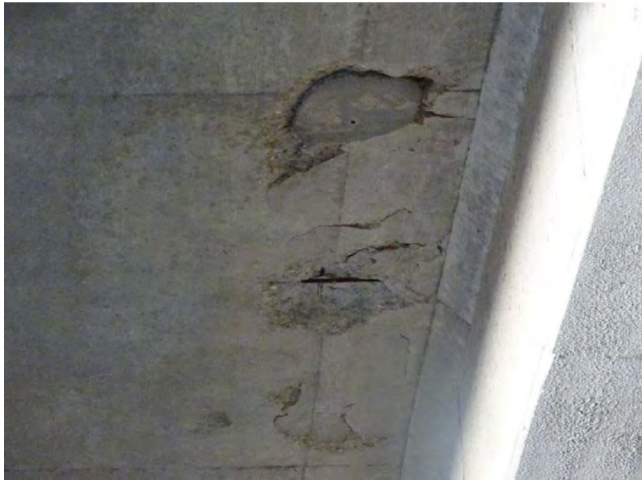
Spall on Bottom of Deck (Typical)
