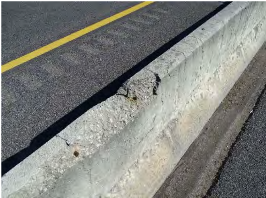
Median Bridge Rail Showing Damage (Typical)
