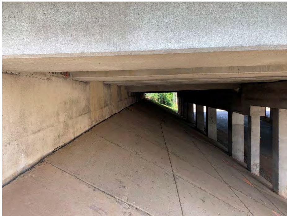
Abutment and Concrete Lined Slope (Typical)
