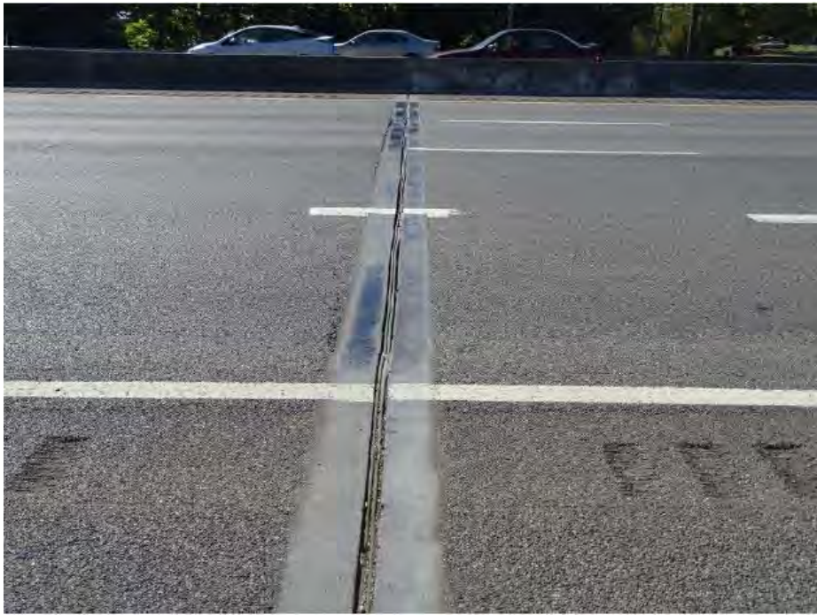
Joint at Abutment (Typical)
