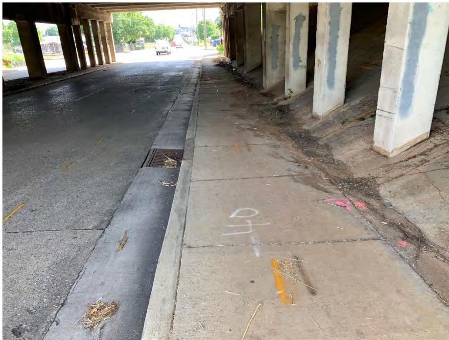
Eastbound Sidewalk Under Span No. 1 Evidence of Poor Drainage
